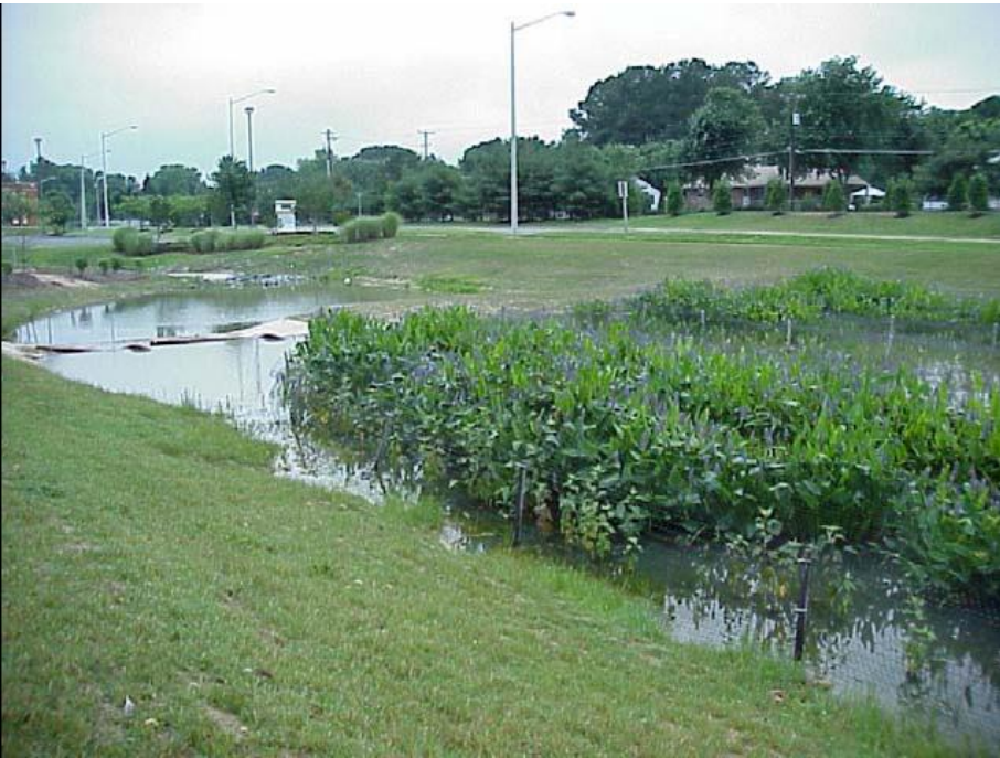
Constructed Stormwater Wetland
